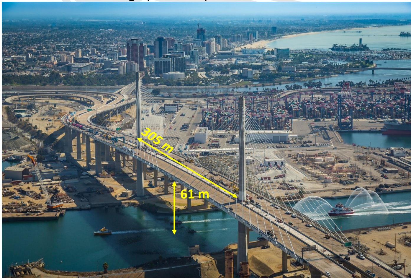
Gerald Desmond Bridge (California)
