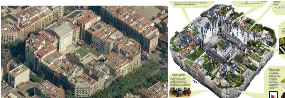
Figure 5.50. Illa Eficient plan for a city block with various proposals for the use of flat roofs, roofs and the interior courtyard.
