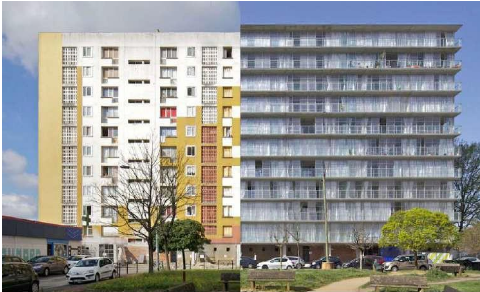
Figure 5.54. Transformation of 530 flats, buildings G, H and I, Grand Parc district - Lacaton & Vassal, Druot, Hutin. Top: Images of the exterior before and after the proposal. Bottom: Images of the space added to the existing volume.
