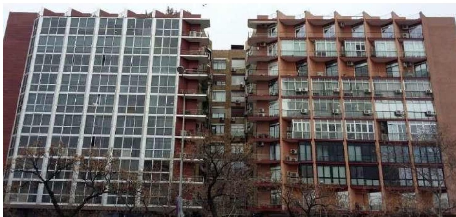
Figure 5.52. View of two buildings with balconies, which were originally symmetrical. The building on the right shows the result of the disorderly enclosure of balconies and the proliferation of heat pumps; the building on the left shows a unitary intervention to renovate the façade.
