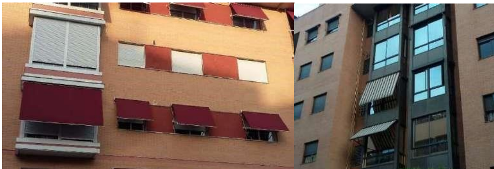
Figure 7.47. Installation of blinds (on the outside) and awnings in glazed enclosed balconies and openings.
