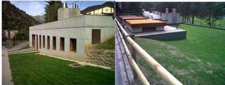
Ribes de Fresser network. Source: Association of Heating and Cooling Network Companies. ADHAC.
