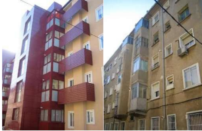
Figure 5.59. Renovation of a building with the installation of a lift on the outside (with the staircase being demolished) and reorganising the clothes drying area. Francisco Franco Group.
