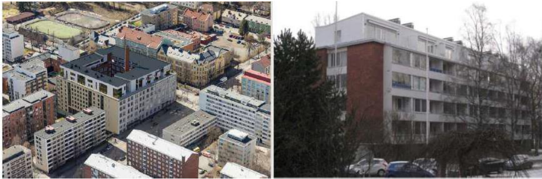
Figure 5.68. Examples of energy renovation with a floor added to a flat roof using a light wooden structure, to contribute to the financing. Rakuunantie, Helsinki.
