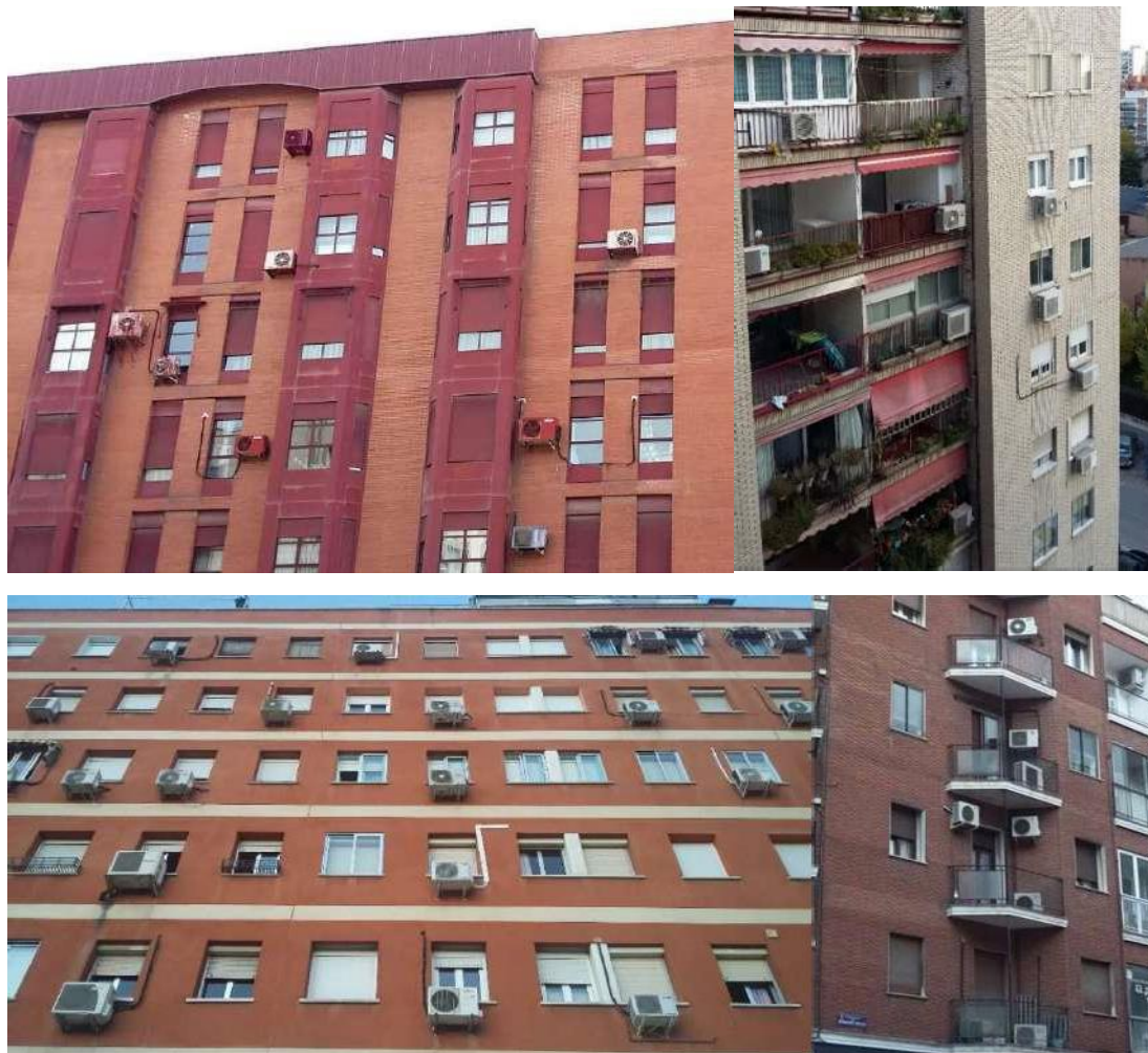
Figure 5.61. Examples of poor integration of heat pumps on residential blocks built between 1960 and 1980.
