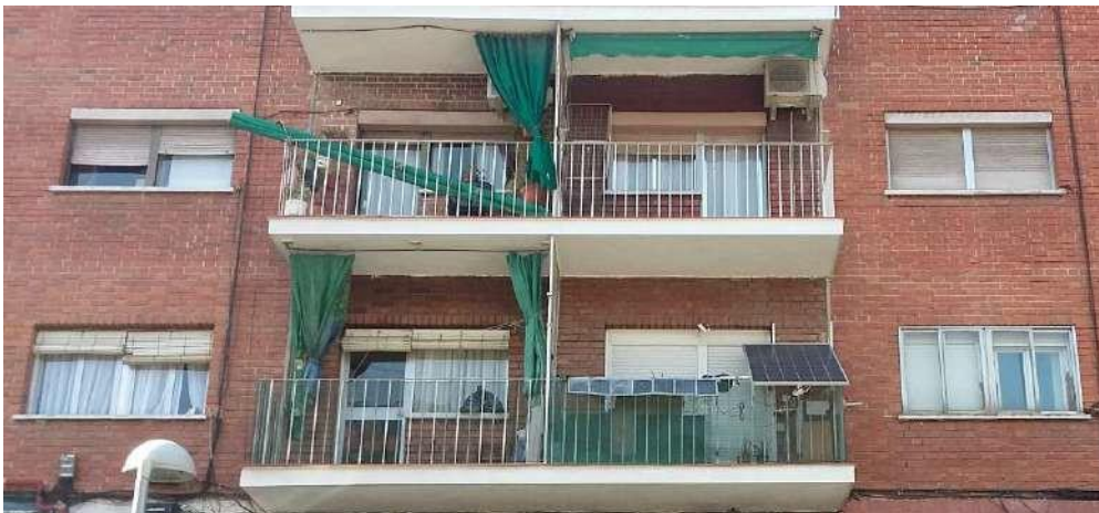
Figure 5.63. Image illustrating the problems relating to the architectural integration of self-consumption equipment in existing multi-family residential buildings.
